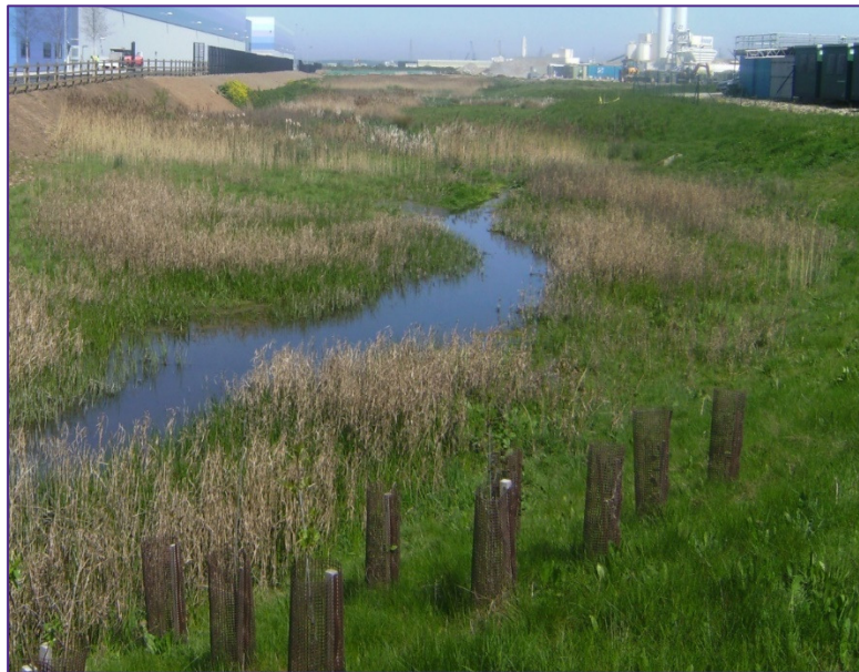
Figure 2-1 Detention Basin with low flow channel
